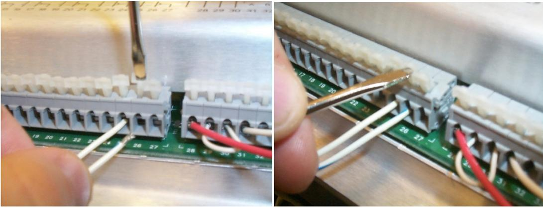
Figure 2-1. Installation of Wiring into Terminal
