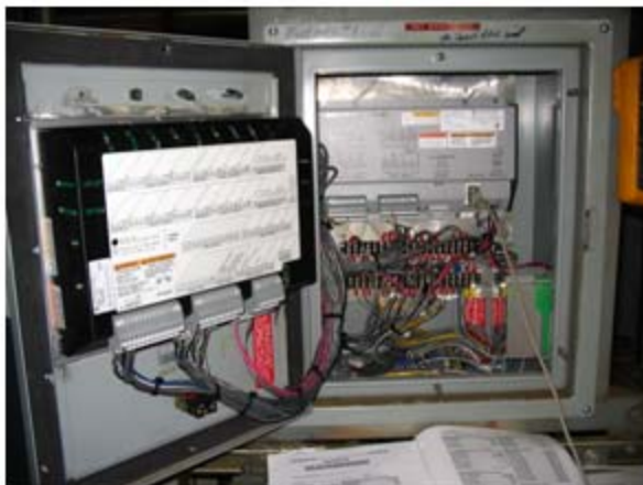
New 505 and SPC Installation in the Original 505 Housing
